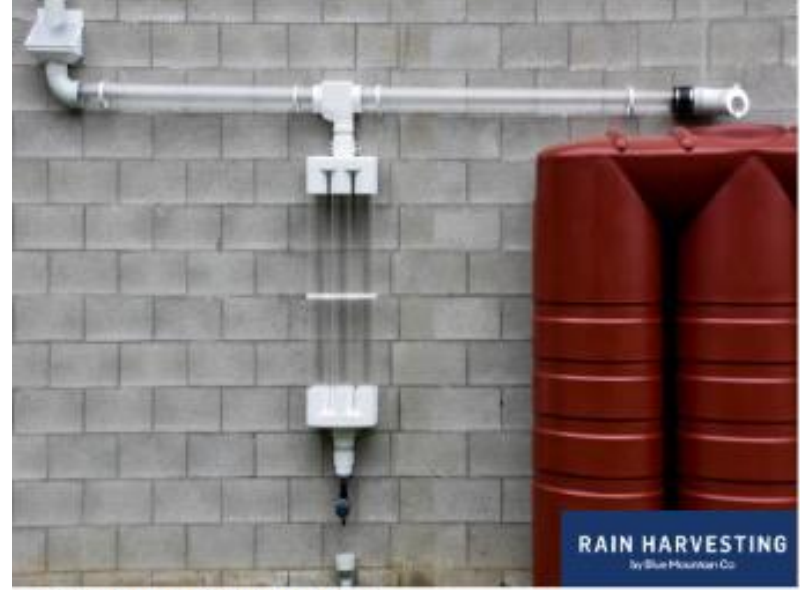
First Flush Diverter
