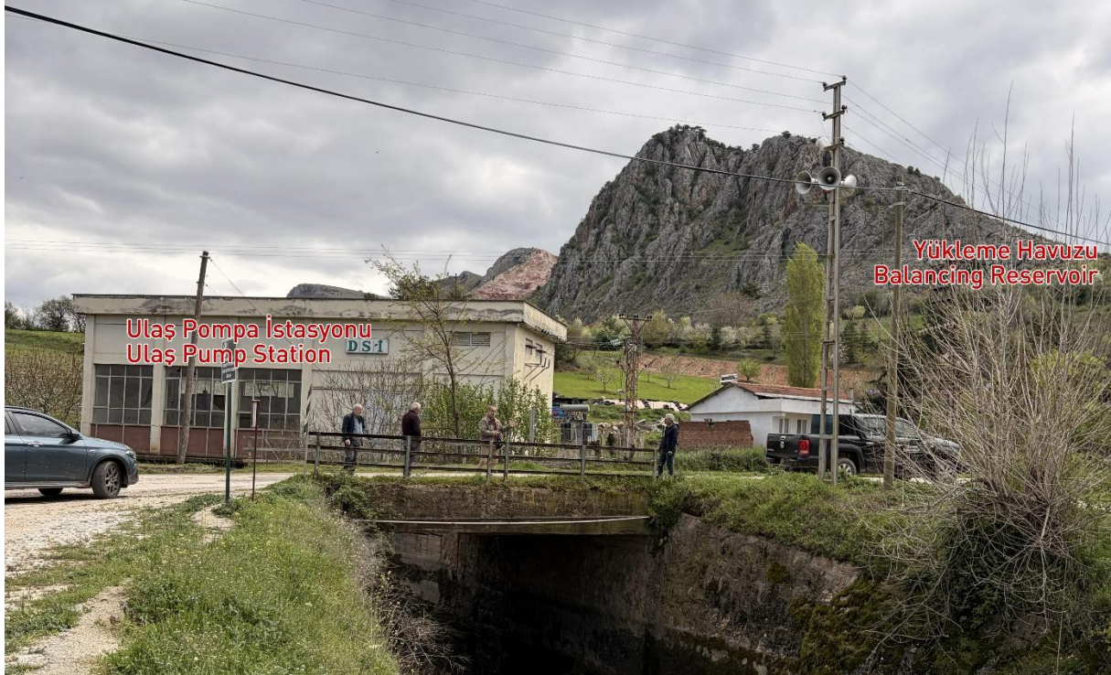
Photograph 3. Approximate Locations of the Proposed Ulaş Pump Station and Balancing Reservoir
