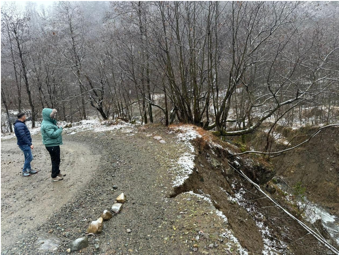
Photo 4: View of the Bölümlü Classical 2 Check Dam Location
