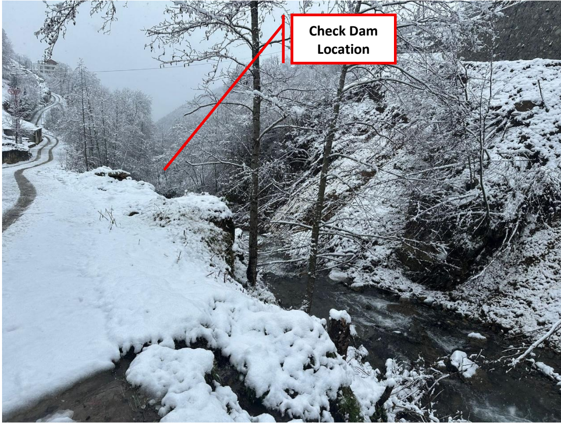
Photo 5: Upper Section View of the Akköse Classical Check Dam Location
