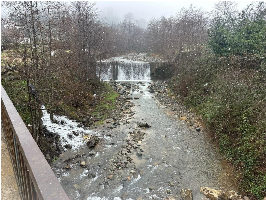
Photo 2. View of the Bölümlü Permeable 2 Check Dam Location
