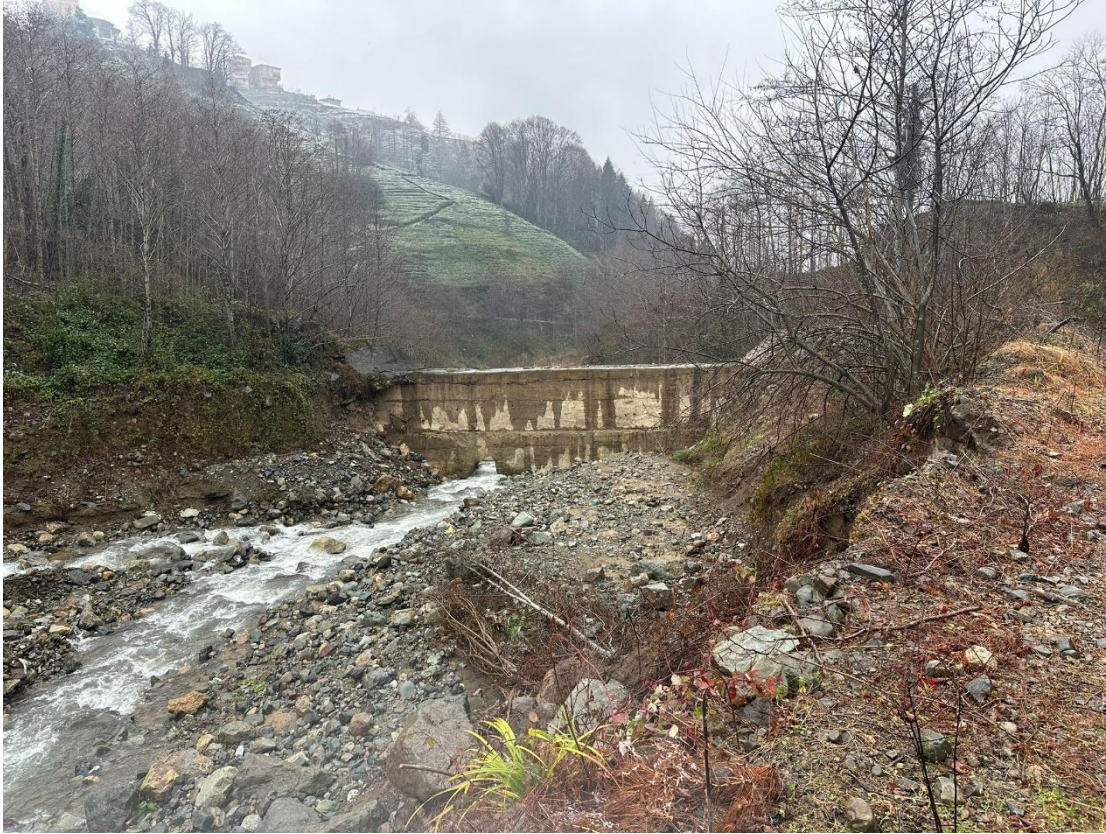
Photo 1. View of the Bölümlü Permeable 1 Check Dam Location
