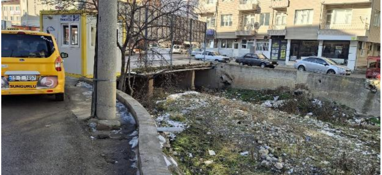
Photo 2-1 General view from the Project Area (Diği Stream)
