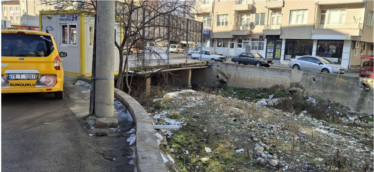
Photo 2-1 General view from the Project Area (Diği Stream)
