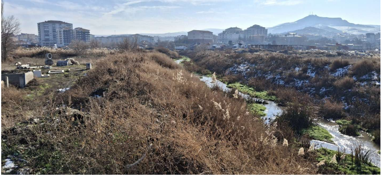
Photo 2-5 General view from the Project Area (Akçay Stream)
