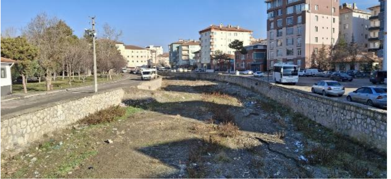
Photo 2-3 General view from the Project Area (Diği Stream)
