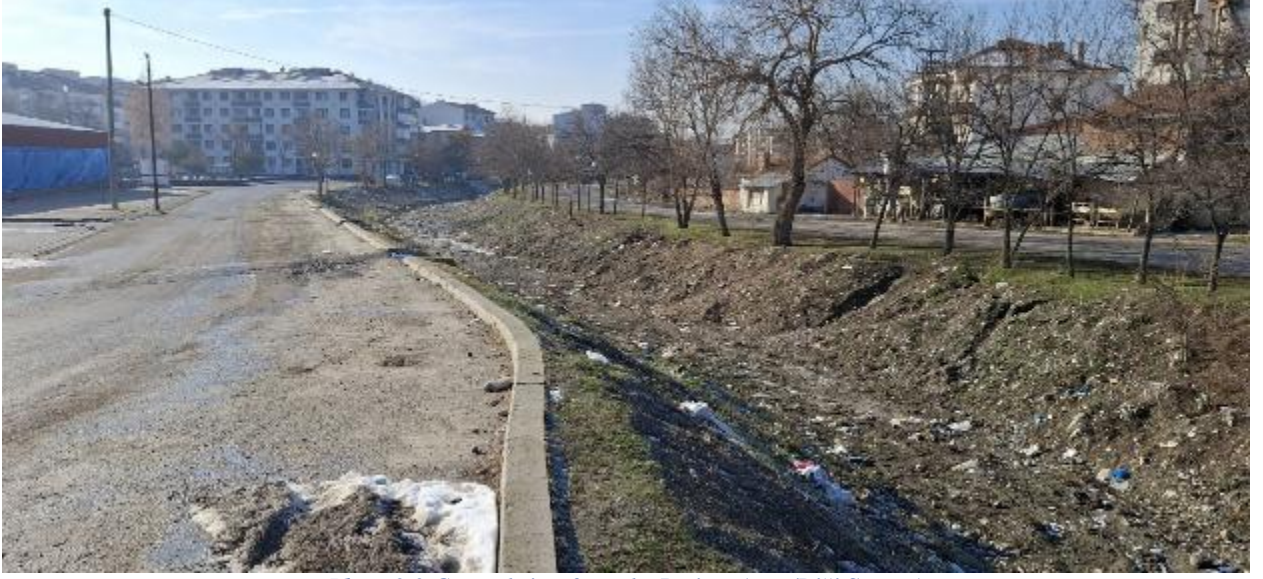
Photo 2-2 General view from the Project Area (Diği Stream)
