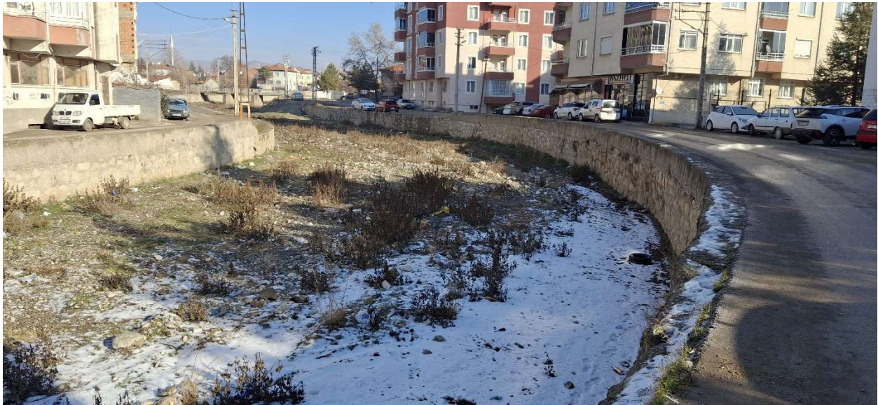
Photo 1-1 General view from the Project Area (Diği Stream)
