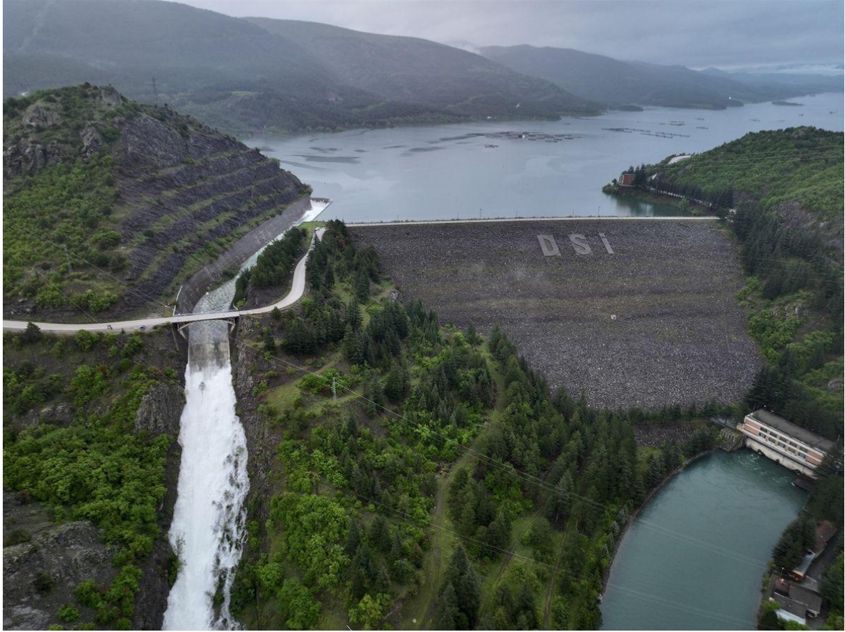
Photograph 8. Almus Dam - General Overview
