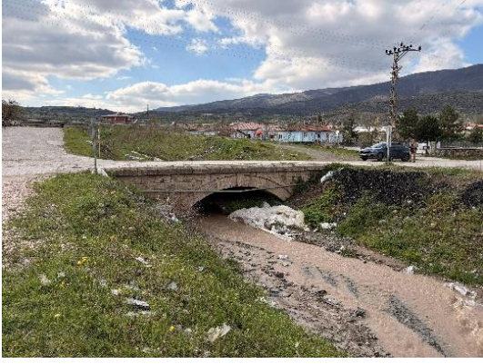
1 - Gümenek Historic Bridge
