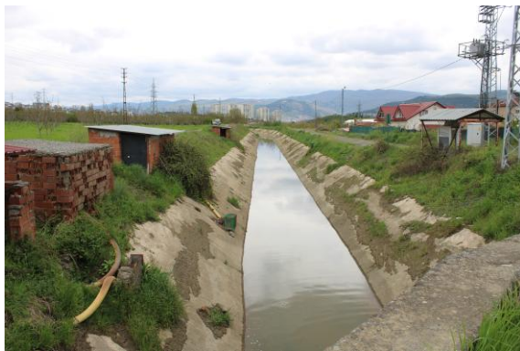
Location of the Pump Station (Approx.)
