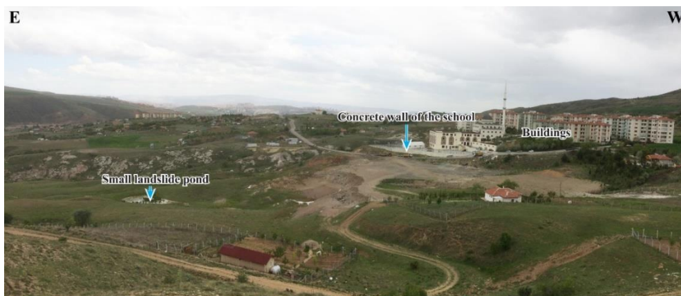
Figure 4 - A view of the landslide (Please refer to Figure 2 for photo direction).
